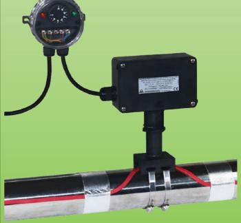
Example of assembly on 3 or more heat tracing cables, in combination with Y25 connection boxes
